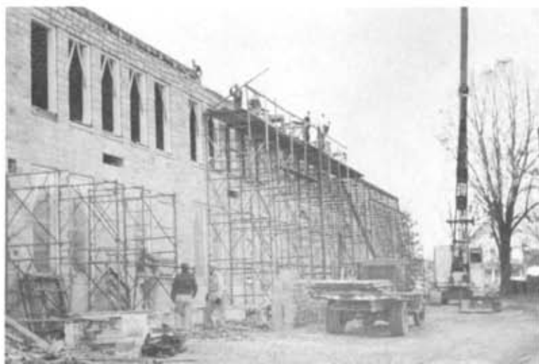
MEN WORKING — VIEW OF NEW ADDITION
